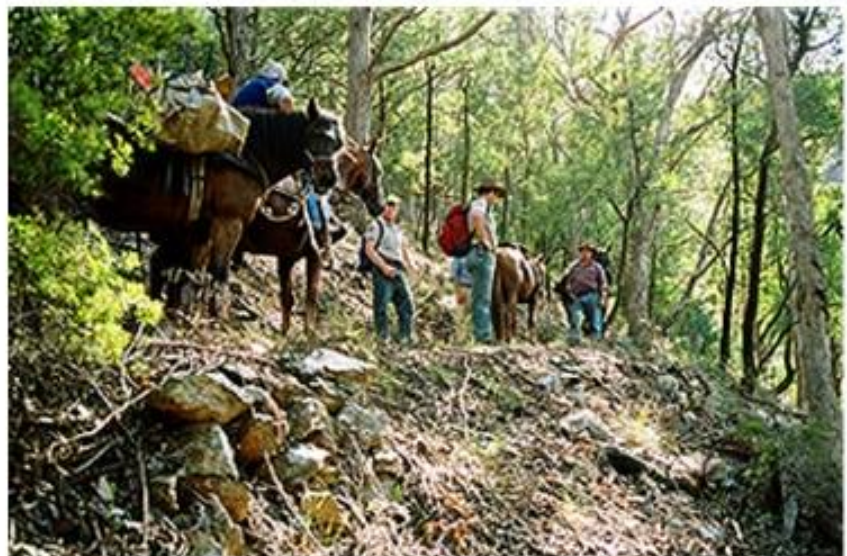
Figure 5 Remnant retaining wall, eastern end, Shoebridge Track, April 2004. PF 2004 photograph
